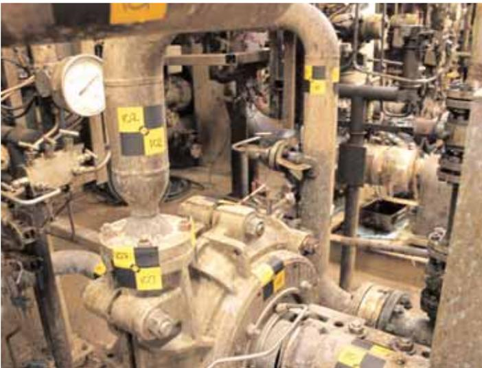
Typical pump layout in an Offshore platform where physical space is limited.
