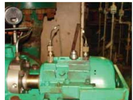
MagTecta-OM-AX™ bearing protectors fitted on a Sulzer MSD2 3x6x9 Model pump.
