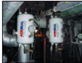
AESSEAL® SSE10™ Barrier Fluid Systems for AESSEAL® CDSA™ Double Mechanical Cartridge Seals in Sodium Silicate Service.
