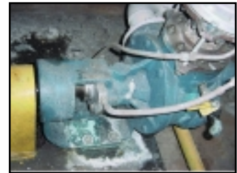
Sodium Silicate Transfer Pump with AESSEAL® CDSA™ in a Viking Pump.
