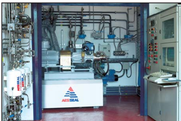
Extensive AESSEAL® test facilities
